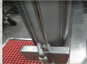
Concealed Pneumatic Control with 316L Stainless Steel Tubing & Fittings
